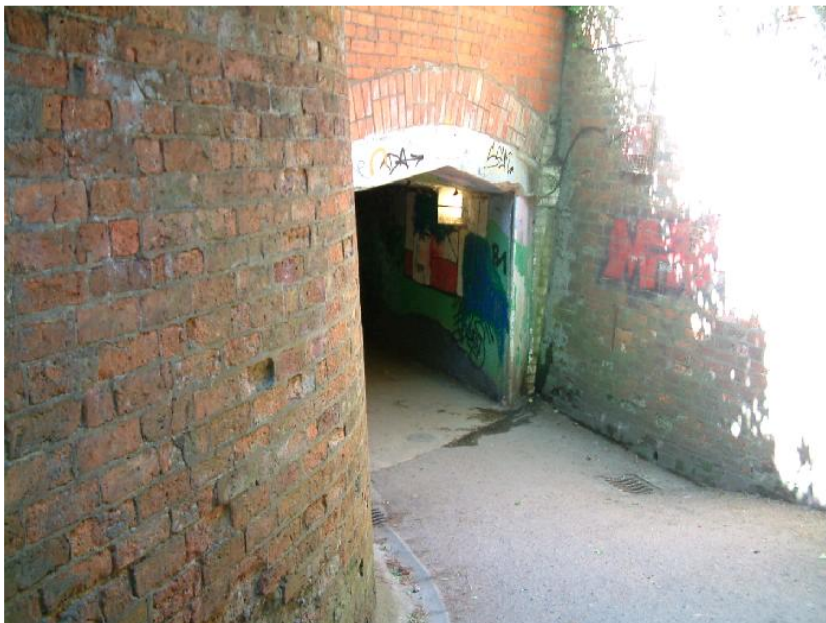
Figure 1: The entrance to the underpass
