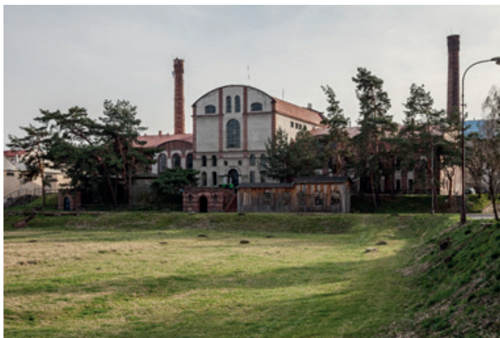
Figure1: Old WWTP, Prague, CZ, The Main Operations Building.
