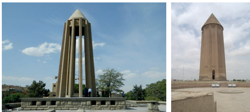
Figure 5. The Avicenna mausoleum in Hamedan (left) and Gonbad-e Qabus tower (right)
