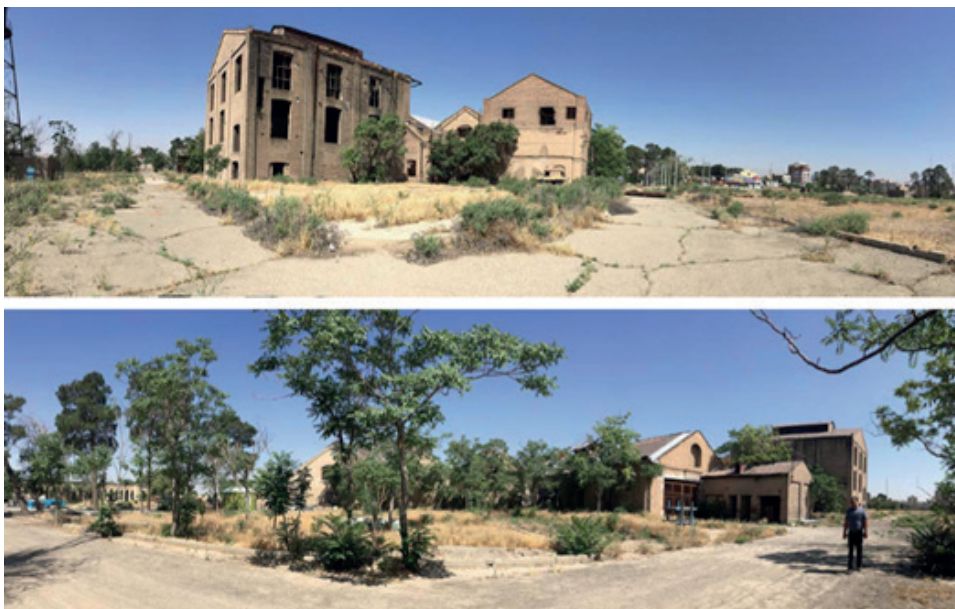
Figure 5 : Full view of Kahrizak sugar factory
