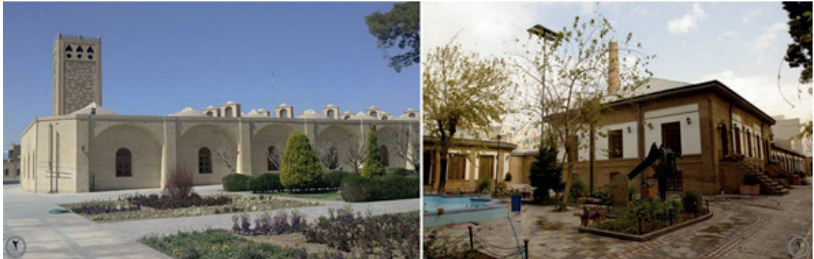
Figure 1. Tehran Stocking(Electricity) Company,area13
