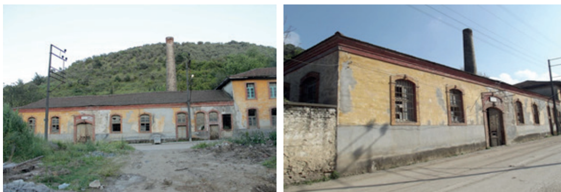
Figure 3. Photographs taken from the main (NW) façade of Tirilye Olive Oil Factory (Acar Bilgin 2015)
