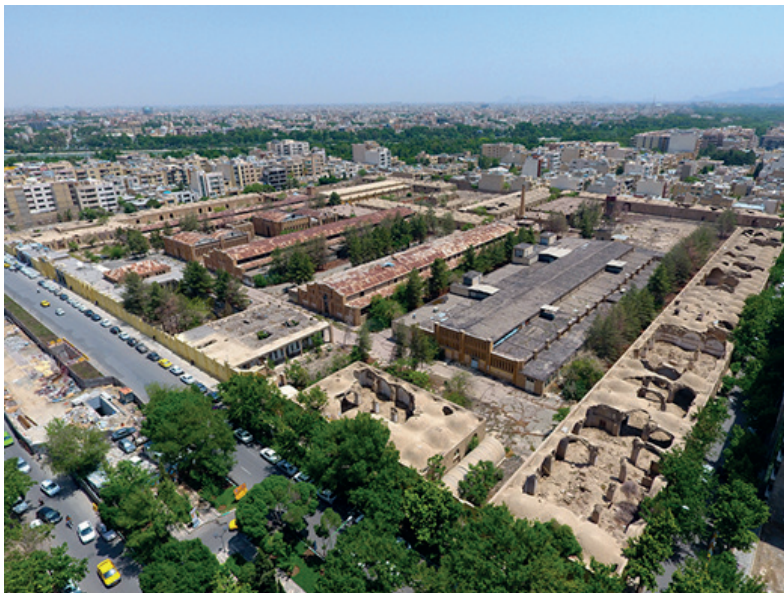
Figure1:Isfahan Risbaf Factory – A large complex housing different industrial, administrative, services, hygiene, and educational functions (Author).
