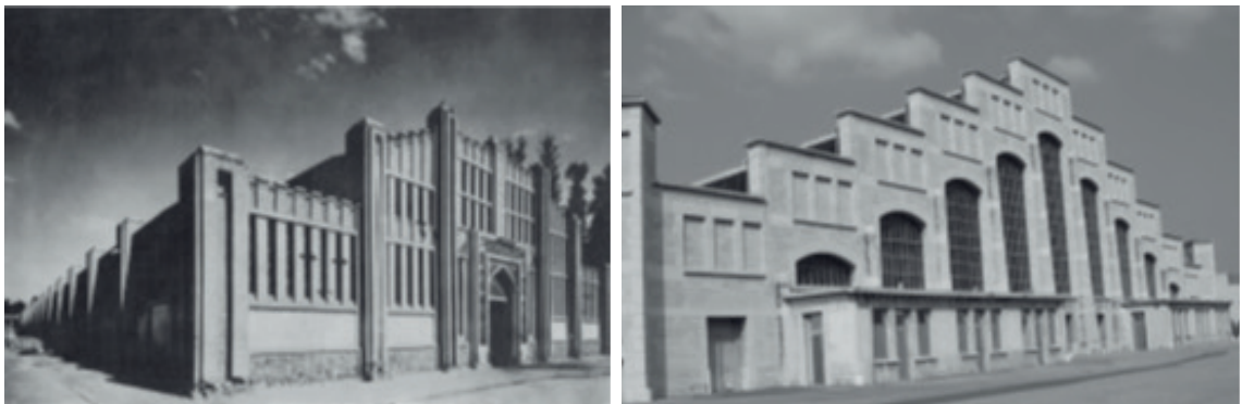
Figure. 4: Pair of images comparing the Risbaf Spinning Factory to the Halle Tony Garnier, Lyon, 1905-1924, by Tony Garnier.
