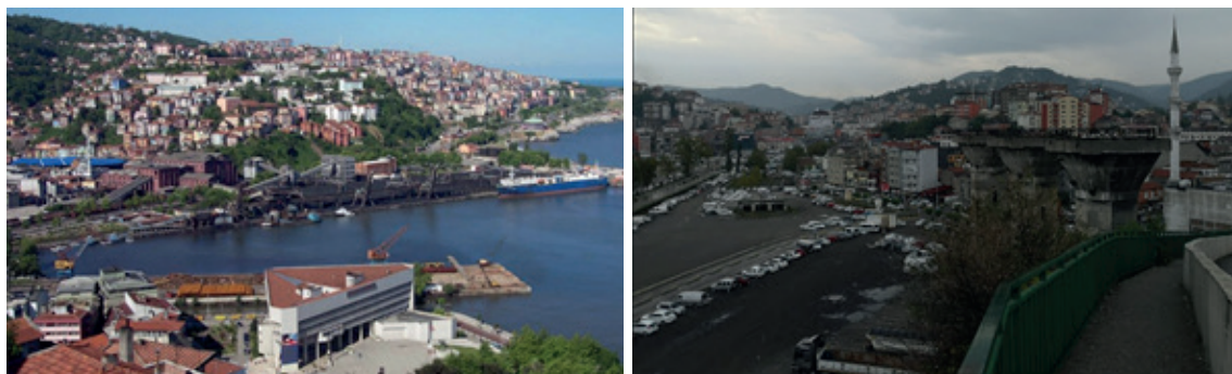
Figure 3. Central coal washing plant before and after the demolitions
