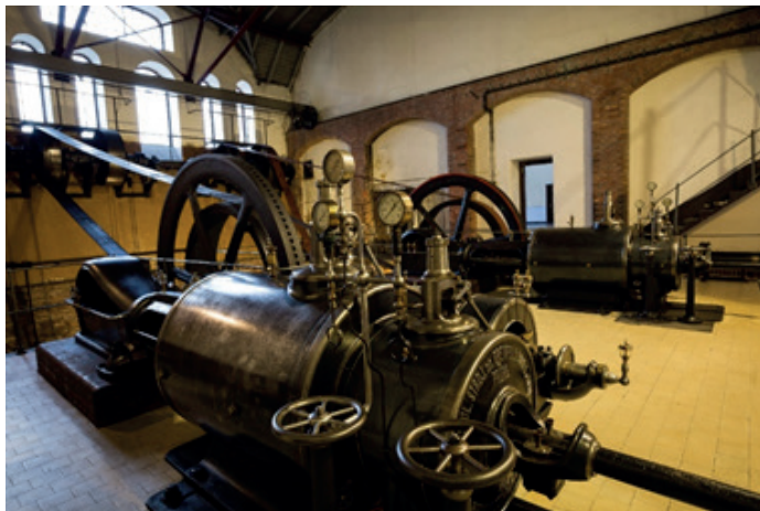
Figure4: Old WWTP, Prague, CZ, The steam engines room.
