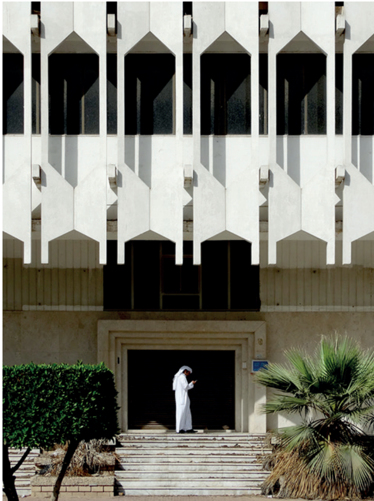
Figure 2. A. Irving, G. Brown, Gulf Bank building, Kuwait City 1963. Detail of the façade (photo R. Fabbri, 2015)
