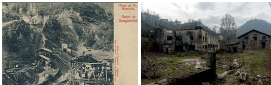
Figure 5. Üzülmez Mines, originally Rombaki Mines, on its first years and today.
