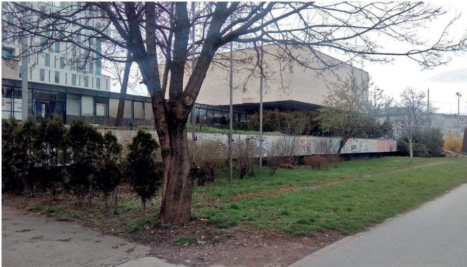
Figure 6: The Museum's state of condition in 2016 4
