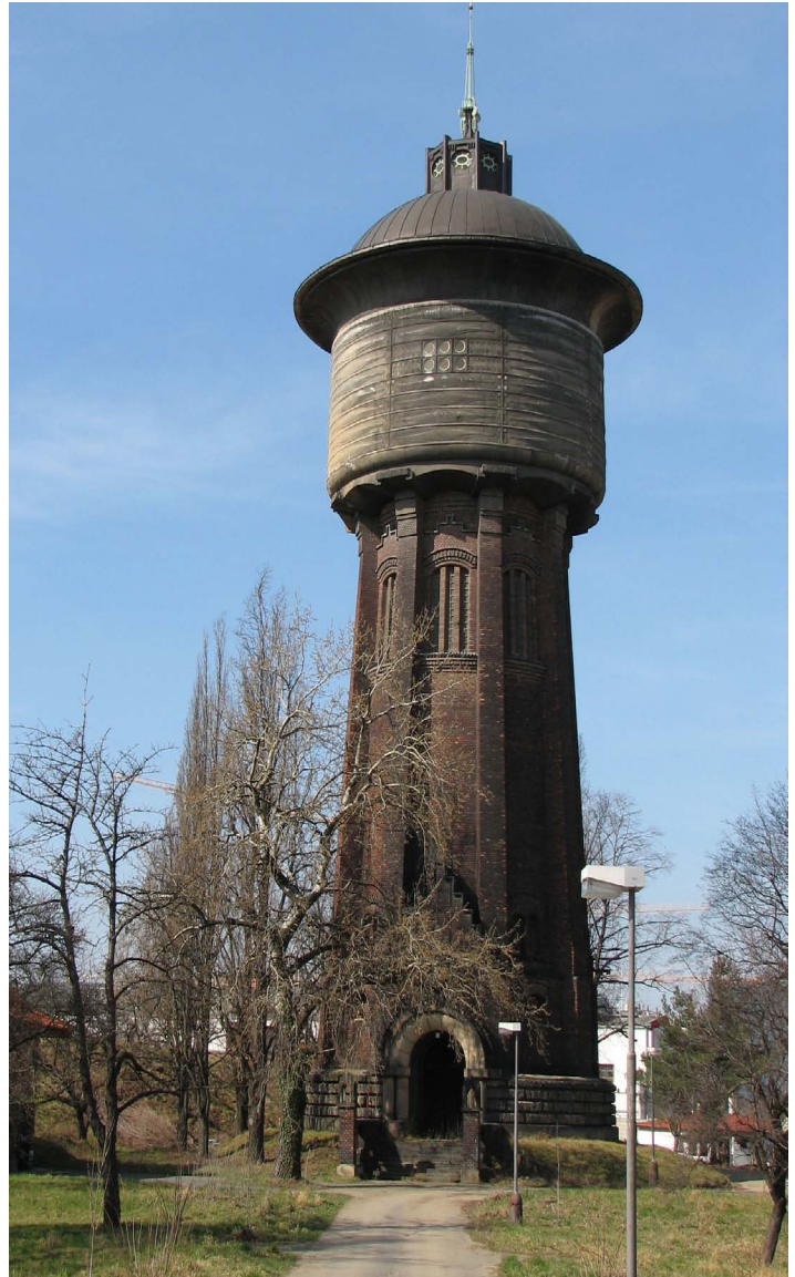
Water tower from 1907, a combination of brickwork and concrete, architectural design by Jan Kotěra ( architecturally important building in the Czech republic), construction by companies K. Kress and B. Hollmann, height 42 meters, steel tank with a volume of 400 cubic meters, the reservoir supplied the territory of Vršovice, later Braník, Krč and Michle.
