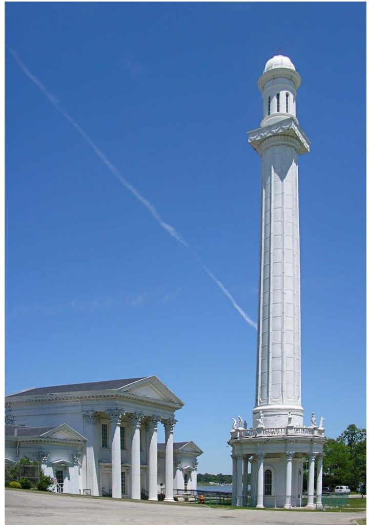
The Neoclassical 1860 pumping station and standpipe of the Louisville, Kentucky, WaterWorks Museum. (Photo: Creative Commons)
