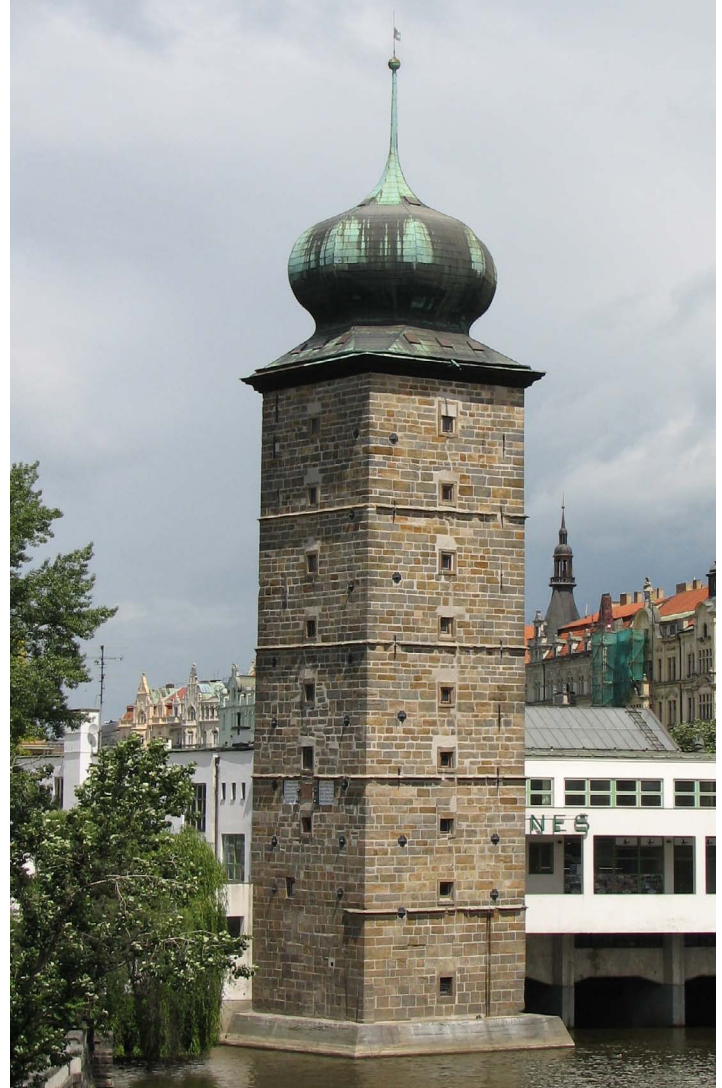
One of the oldest tower reservoirs in the Czech Republic, a building from quarry stone, built in 1588-1592, supplied water from the Vltava River to the New Town of Prague, in 1648 very damaged during the war, it served until 1881, height 47 meters, is deflected from the vertical axis about 42 centimeters, in the past in the upper part of the tower water reservoir with a volume of 2 cubic meters.
