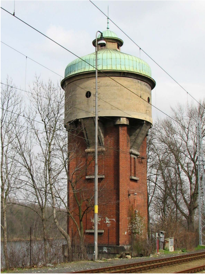
The water reservoir built in 1927 by A. Hádl and F. Hájek, utilization for the railway station Roudnice (supply of steam locomotives with water), reinforced concrete structure with brick masonry, two reinforced concrete reservoirs (total volume of 120 cubic meters).
