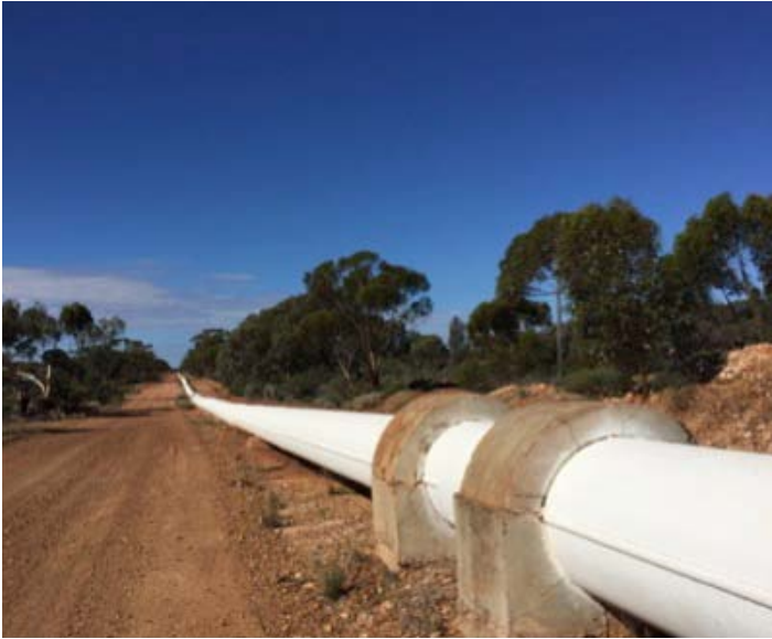
The Goldfields 'Golden' Pipeline (Photograph: Dr Nina Hall)
