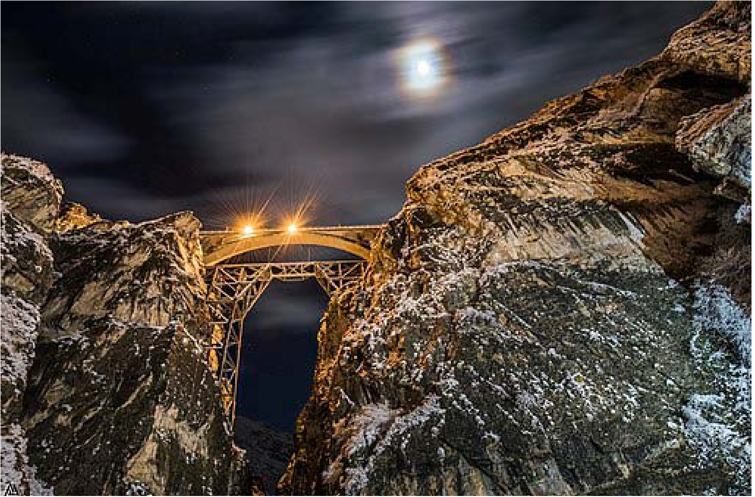
The famous Veresk bridge has a 66 m span and a height of 110 m and was built without using any metal materials or armature. Photo: Ahmad Jamali M, 2017
