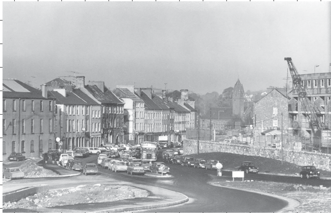
Photo documenting the demolition caused by the construction of the Newry Through-pass in the early 1970s. Image source: Newry and Mourne Museum Collection, NMD Museums.
