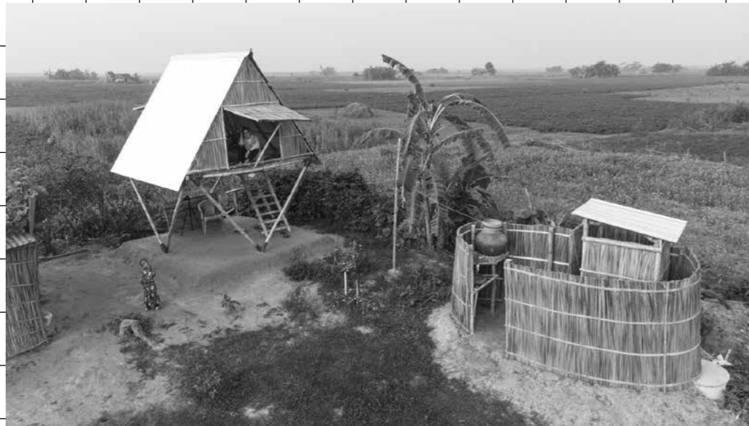
Photograph of a housing system of mobile modular structures made from bamboo; Khudi Bari. Photographed by Asif Salman.
