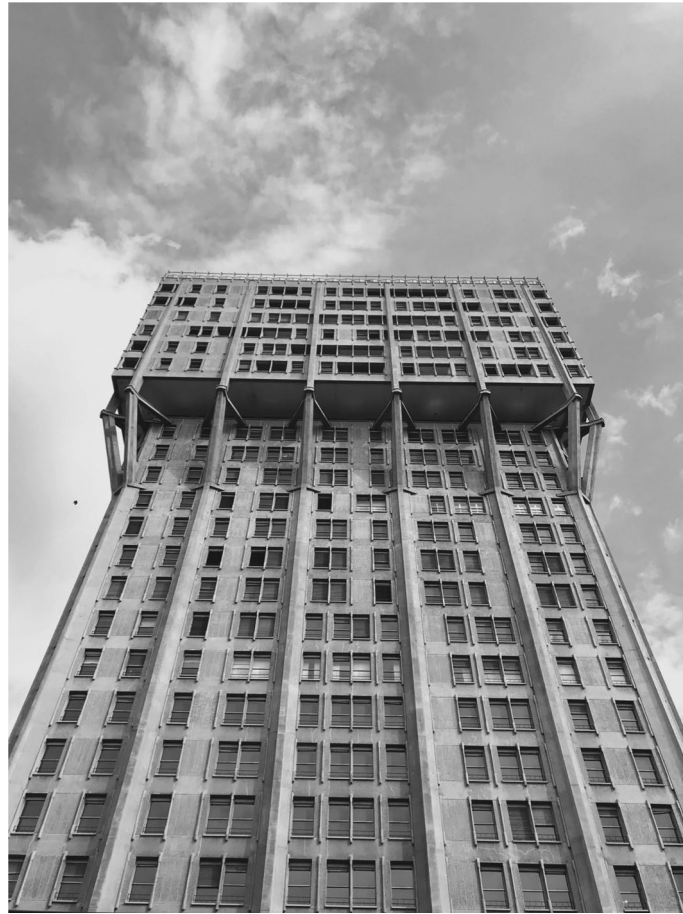
Fig. 11 Torre Velasca (1950–8) by Ludovico Belgiojoso, Enrico Peressutti and Ernesto Nathan Rogers (BBPR). Photograph taken by Marianna Charitonidou, 13 June 2018
