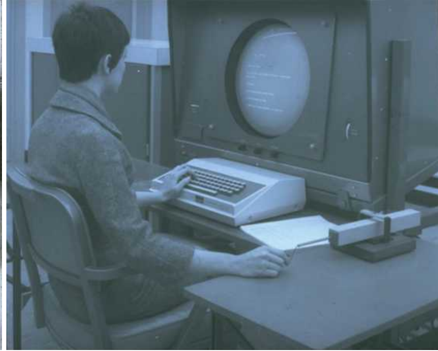
Augmentation Research Center: Left: A knee-operating pointing device as an alternative to a mouse, 1967 or earlier. Right: Grafacon, movable gyro-style pointing device as an alternative to a mouse, c. 1965.
