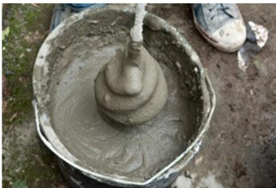
Fig.4 Mixing the adhesive Source: howtospecialist.com
