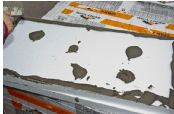
Fig.5 Applying the adhesive. Source:howtospecialist.com
