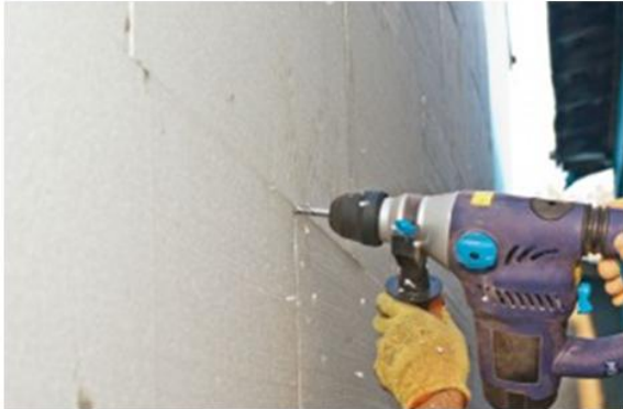
Fig.6 Securing the (EPS). Source:howtospecialist.com
