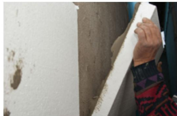
Fig.5 Installing the (EPS). Source:howtospecialist.com
