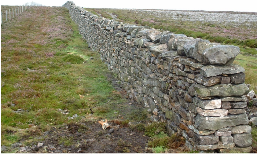
Figure 3.2 Dry stone wall in Donegal Med Partnership, Creative Commons license.
