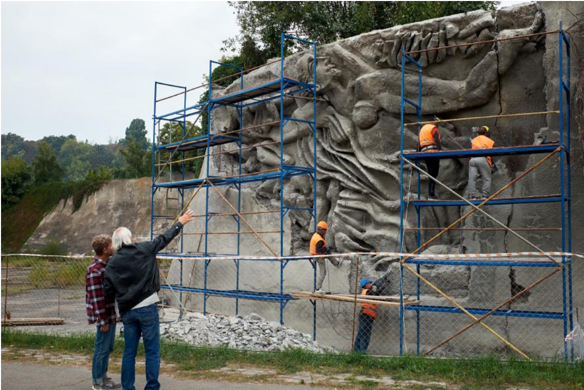
Figure 30. The Wall of Remembrance in the Baikove Cemetery took ten years to build, yet in 1982, when it was finally complete, authorities decided to plaster over it. Today, various methods are being employed to remove the concrete and uncover the reliefs hidden underneath. [Fujifilm X100F, ISO 800, f /5.6, 1/900; September 17, 2021]
