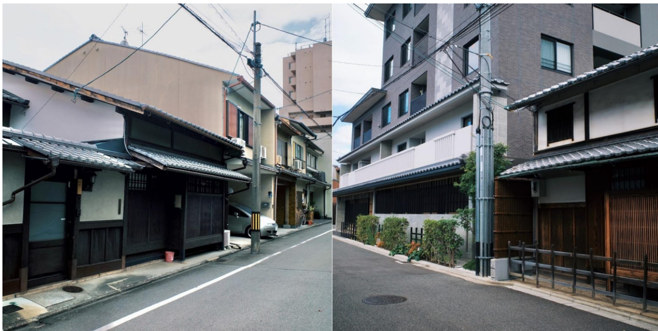
Figure 1: Machiya in the Kyoto neighborhood of Nishijin. At left, a traditional machiya sits alongside more recently built homes that refer to the same vernacular. At right, a modern apartment building, which features tiling, eaves, and latticework in the same vernacular, sits next to an old machiya. Photos by the author.
