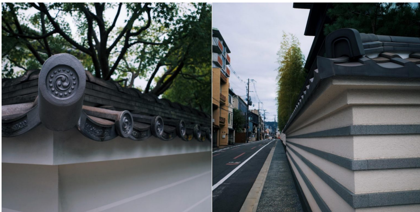
Figure 2: The wall of Myōkenji temple in the Kyoto neighborhood of Nishijin, at left, and the wall of The Mitsui Kyoto—a modern hotel south of Nishijin, at right, both use the ichimonji-gawara (single-line tiling) style. Photos by the author.
