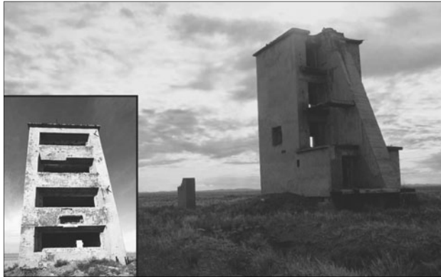
Figure 6: Front (left) and rear (right) views from 2013 of a reinforced concrete scientific station at the former Soviet nuclear weapons testing site at Semipalatinsk in Kazakhstan.
