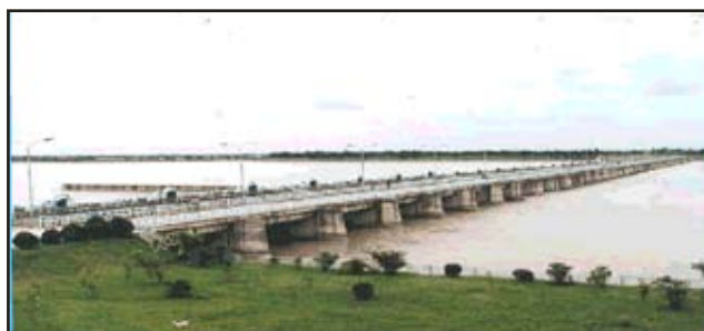
Figure 1: A view of the Dalia Barrage, Bangladesh.
