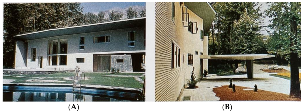
Figure 6. (A) The South-facing villa façade seen from the pool, showing double height reception window at the left, and entrance to the interior courtyard on the right. (B) Photo of the front façade with the elongated canopy entrance supported by a diamond-shaped pier. The villa was covered in Ponti's "Diamanti" tiles made by Ceramica Joo. Source: [1] (pp. 14–19) also, seen in [6] (p. 324).
