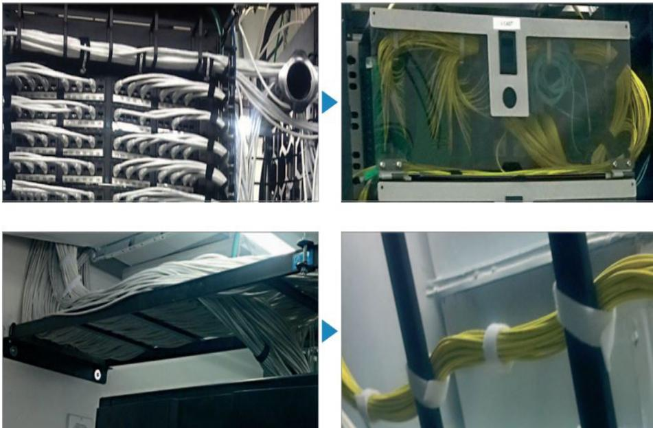
*Figure 7.* Cable size of CAT 5 vs. optical fiber Implemented in the same building infrastructure. The rack and cables at the left side were an early LAN implementation supporting one half floor. The yellow cables at the right side are the Passive Optical LAN implementation to replace the original LAN implementation—supporting three and one half floors.
