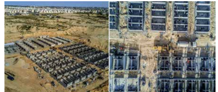
Figure (5): Construction of a field hospital in Rafah, Gaza Strip. 19
