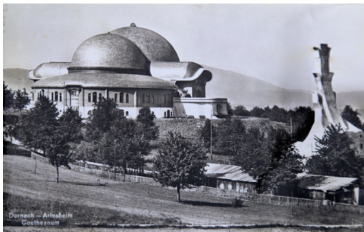
Fig.6. The Goetheanum, Foundation Stone laid 20 September 1913, opened on 26 September 1920, destroyed by fire 31 December 1922 (Paull, 2020).
