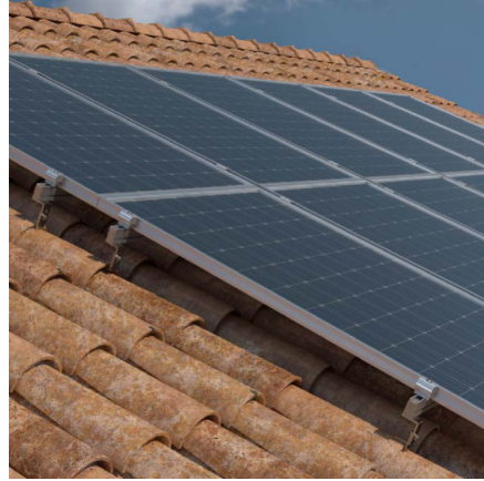
Figure 7: Alternative solution: solar panels overlapping the existing roof, allowing the integrity of the roof and its traditional materials to be preserved with a very modest elevation of the whole.
