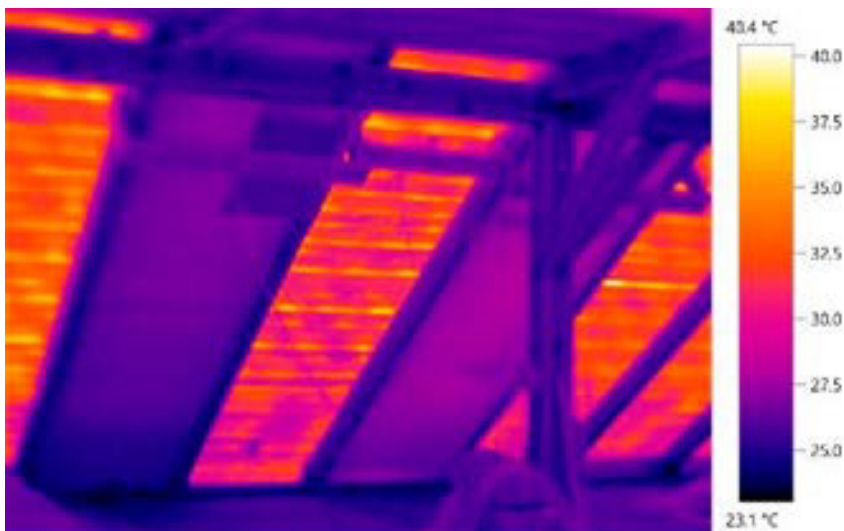
Figure 6: Infrared shading Stadel Bad Goisern. Thermography Günther Kain.
