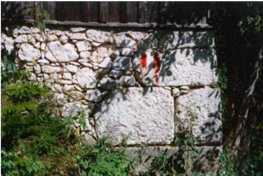
Figure 5: Plinth masonry of the Schafferstadel Hallstatt. Photo Friedrich Idam.
