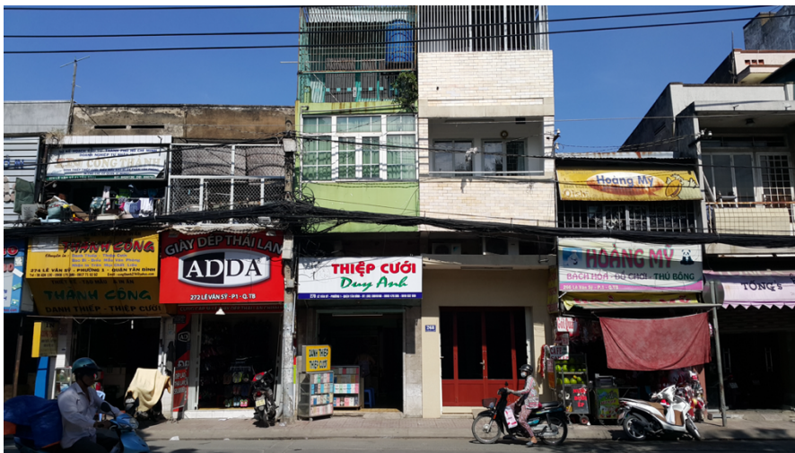
Figure 50. Burglar Proof Windows on Row Houses in HCMC
