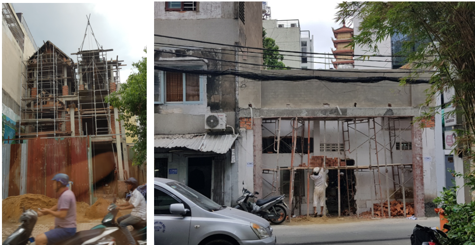
Figure 37. Construction of Self-built Housing in HCMC
