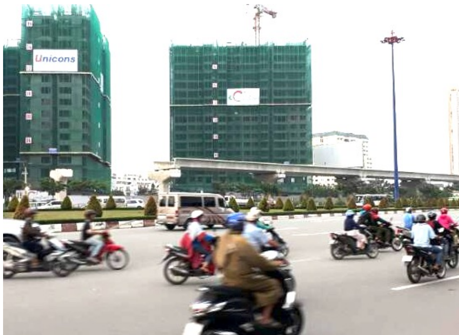
Figure 53. Construction of Apartments and Elevated Metro Railway in HCMC
