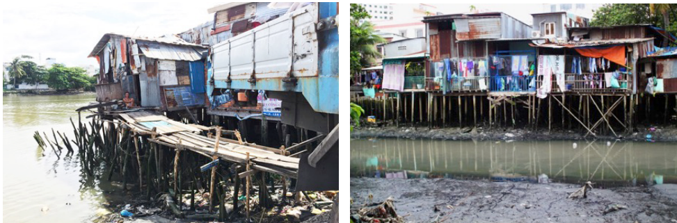
Figure 35. Temporary and Dilapidated Houses in HCMC Source: UN Habitat, 2008
