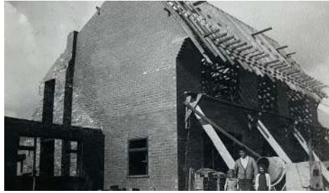
The Construction of 222 Longmeanygate (circa 1966).
