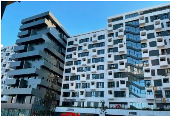
Alpolic panel installed in the façade ( Source: Authors)
