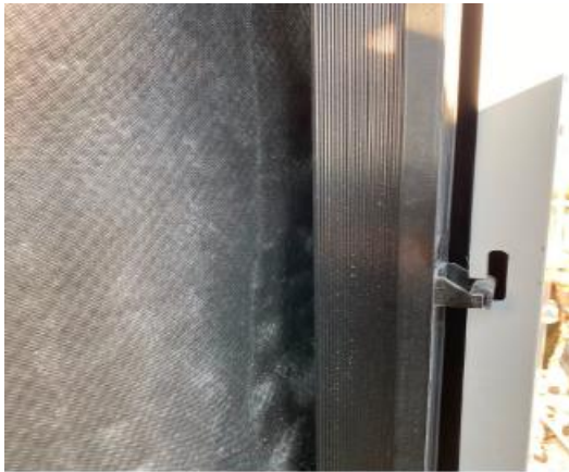
Fig. 5.B- Detail of Alpolic installation ( Source: Authors)
