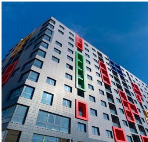
Fig. 5.D- Durabond panel installed in the façade ( Source: Authors)
