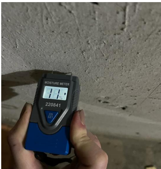
Fig. 4. Measure meter on concrete wall with Admixture.
