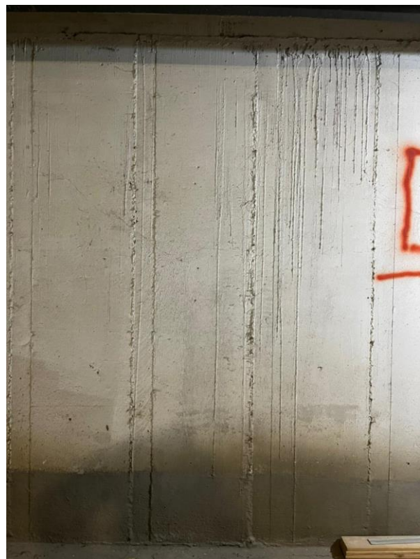
Fig. 7. No visible Moisture on concrete wall with Admixture.
