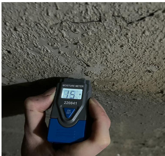
Fig. 5. Measure meter on concrete wall without Admixture.
