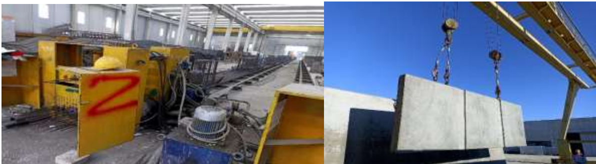
Figure 3. Factory production and concrete transportation; Source: authors
