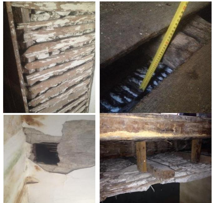
Fig. 4. A. Wooden indoor partition wall; B. Wooden slab; C. Bottom cover of the wooden slab; D. Section of the wooden slab
