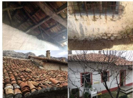
Fig. 5. A. Wooden roof; B. Outer stone wall; C. Ceramic tiles of the roof; D. Concrete pavement connected to the ground floor
