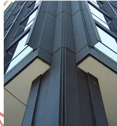
Fig 3: Lake Shore Drive Apartments (Mies Van De Rohe)
