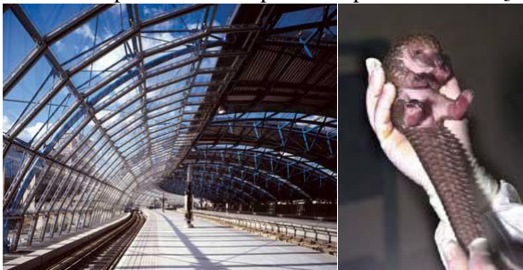
Fig 12: Nicholas Grimshaw & Partners' Waterloo International Terminal and the pangolin.
