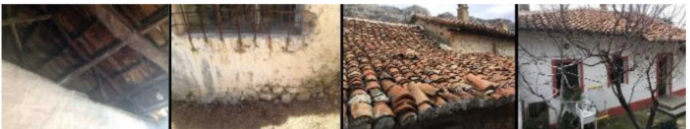
Fig.5 A characteristic dwelling in Kruja citadel. A. Ceramic Roof tiles; B. Stone wall in direct contact with the terrain; C. Ceramic tiles covering the roof; D. Additional concrete pavement for moisture protection. Source: Author
