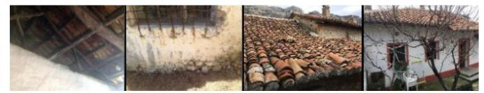
Fig.5 A characteristic dwelling in Kruja citadel. A. Ceramic Roof tiles; B. Stone wall in direct contact with the terrain; C. Ceramic tiles covering the roof; D. Additional concrete pavement for moisture protection. Source: Author
