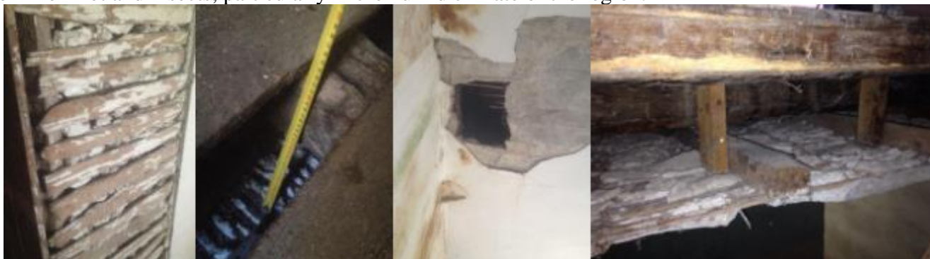
Fig. 6 A. Detail of the partition wall made with a wooden structure and plaster; B. Dimensioning of the wooden soffit (25-30cm); C. Detail of the ceiling closure with reeds + plaster; D. Wooden ceiling cutout. Source: Author
