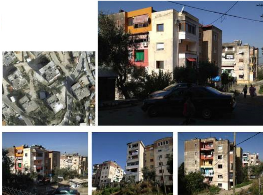
Figure 9A. Socialist building dating from the second half of the XX century, Photos of the existing situation; Klodjan Xhexhi
