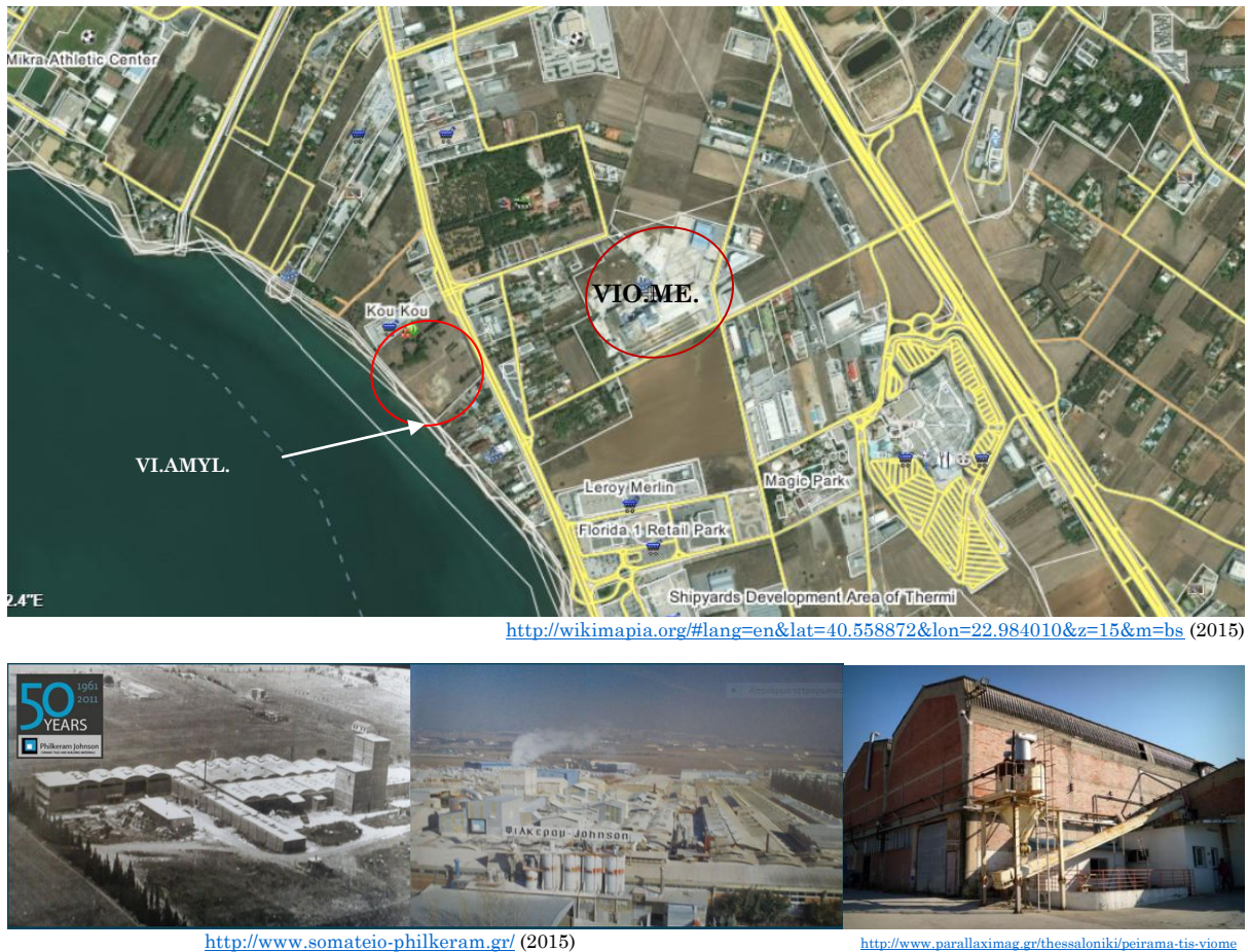
Fig. 6 The Philkeram-Johnson S.A. – VIO.ME. industrial complex, Thessaloniki, GR – location, buildings
