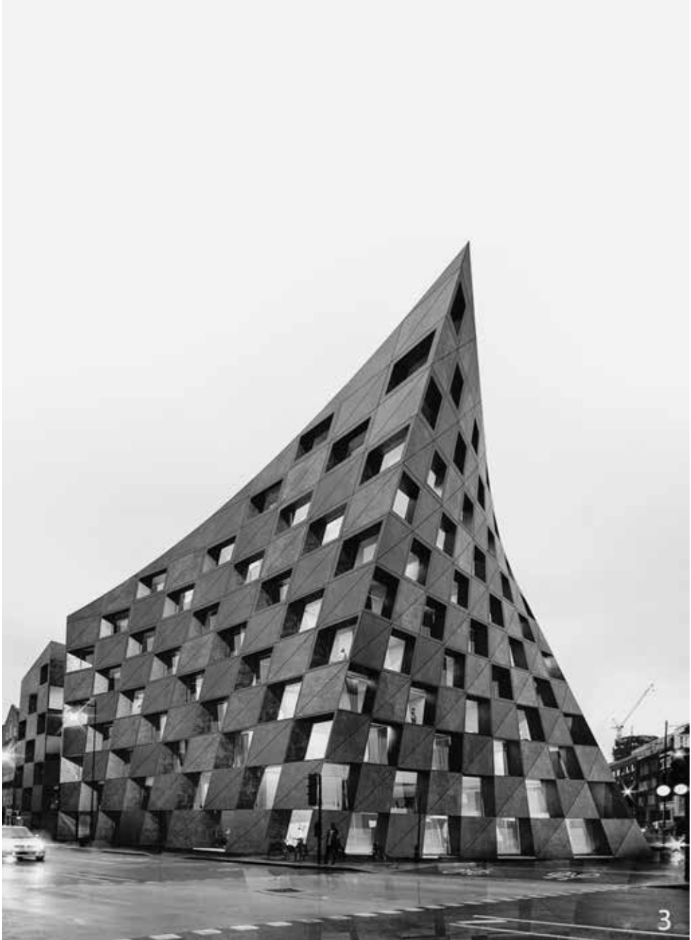
III. 3. AQS Arquitectos, Shoreditch Hotel , London, 2017 http://www.archdaily.com/ (access: 2.5.2020)
