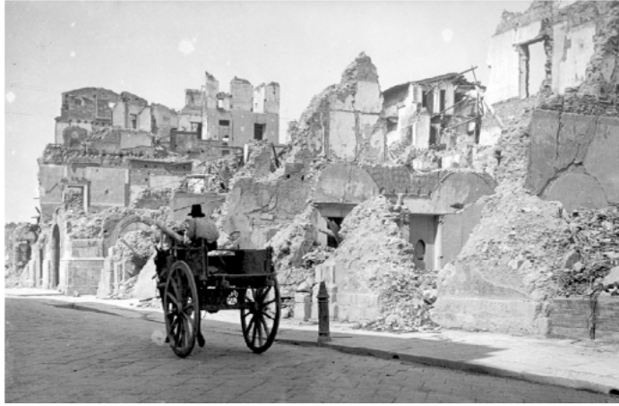
Figure 3 A street in Messina, after the earthquake, 1908
