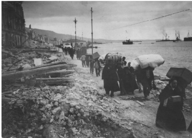
Figure 2 Messina's harbour, after the earthquake, 1908
