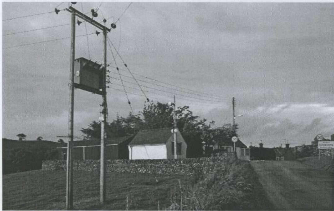
Figure 26.7 Rural telephone exchange, Dunscore, Dumfriesshire, 2002. This telephone exchange is a very modest presence in the landscape for a service which revolutionised communications to, from and within the countryside. SLA 0671.
