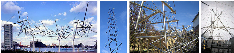
Figure 2 Tensegrity structures: three K. Snelson's sculptures, mast with tensile membrane
